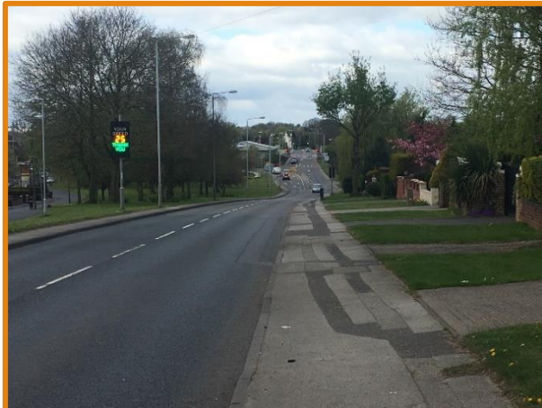
Photograph 3: footways on both sides of Newark Road (looking west from Searby Road)
