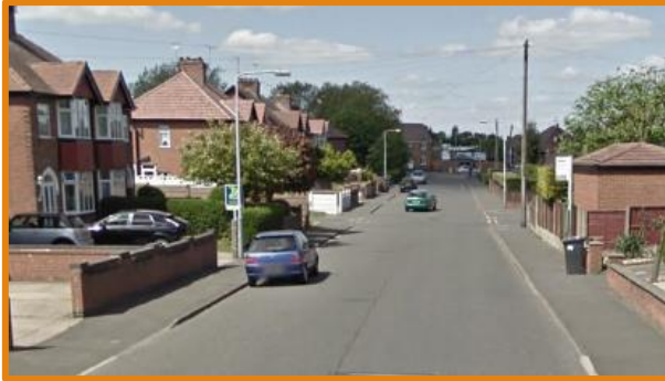
Photograph 5: footways on Farndon Road
