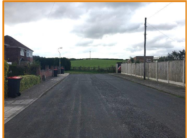
Photograph 4: footways on Searby Road (looking south towards site)
