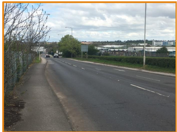
Photograph 2: footways on both sides of Coxmoor Road (N) (looking north)
