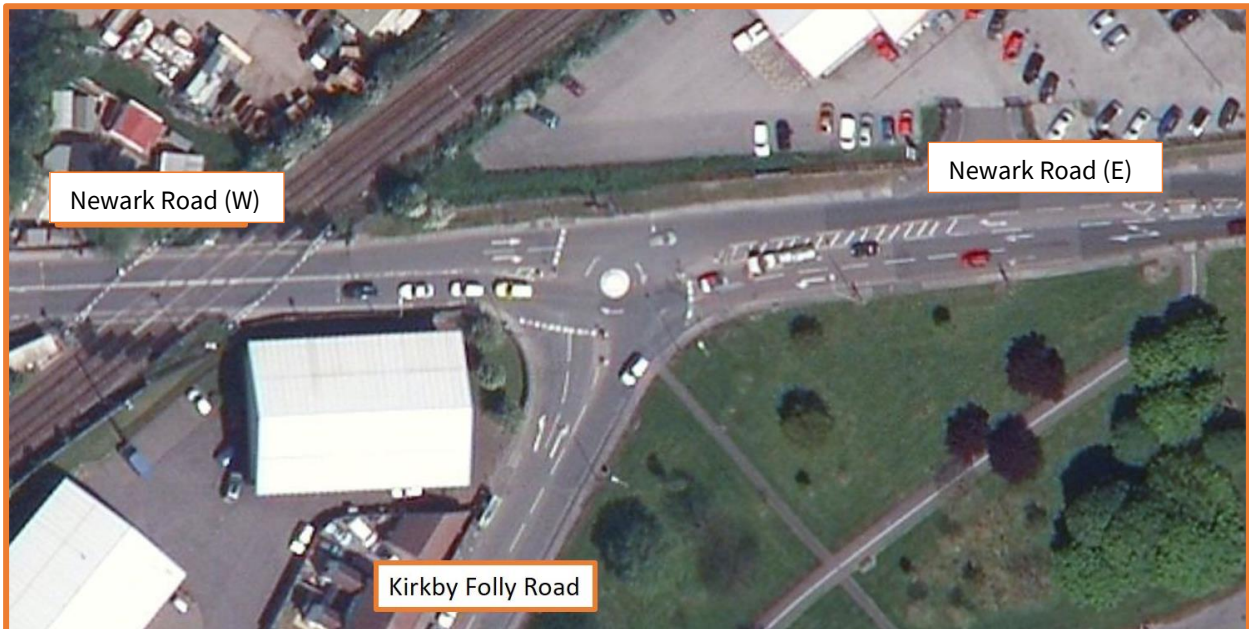
Figure 17: existing Newark Road/Kirkby Folly Road mini-roundabout
