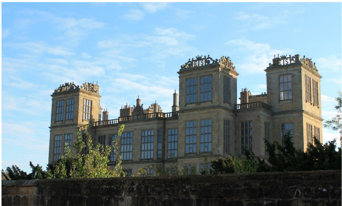
Figure 2. Hardwick Hall, West Front beyond the forecourt wall
