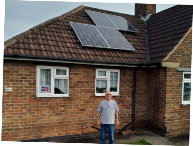
Huthwaite tenant benefiting from new solar panels
