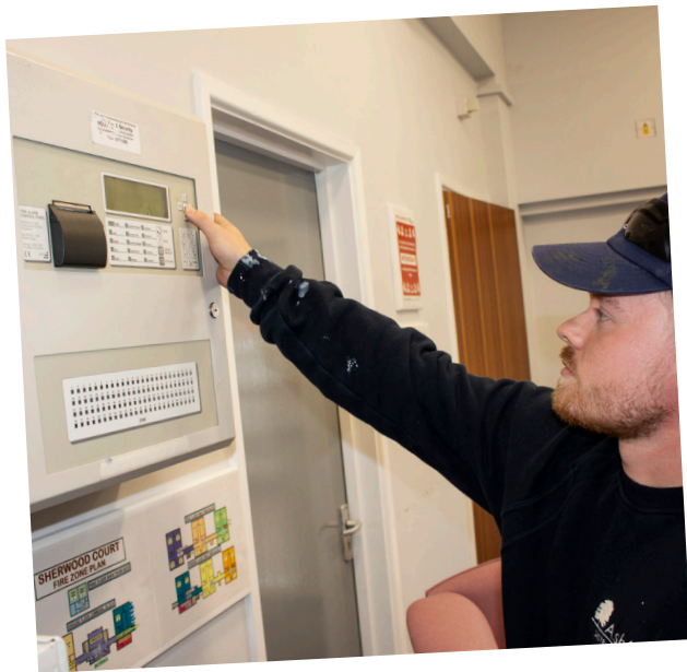
Housing repair technician inspecting a fire board
