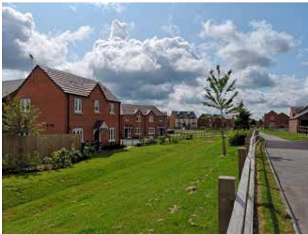
The Larwood residential development in Kirkby-in-Ashfield. With kind permission of W Westerman Ltd.
