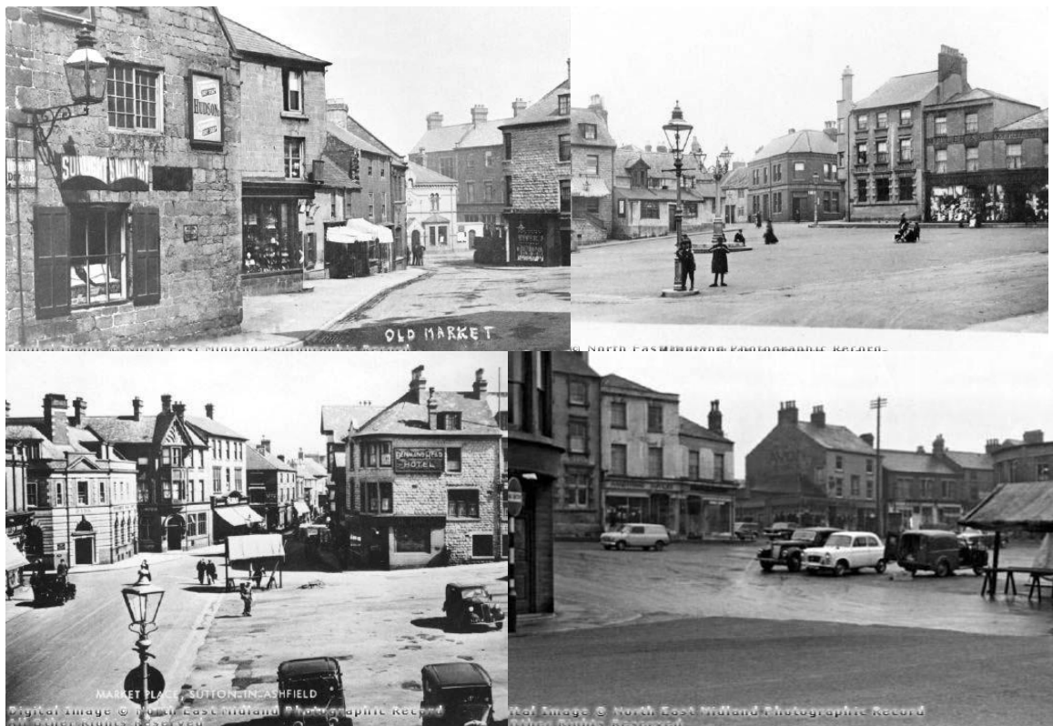
Figure 38: Top left, the Market Place c 1900 before the demolition of buildings on King Street. Top right, the new Market Place shortly after 1905. Bottom left; Market Place 1930s, note the defined carriageway of the road and the moveable stalls. Bottom right; Market Place in the 1960s still being used for car parking as well as trading.
