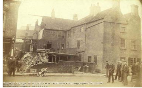
Figure 17 The Denman's Head during rebuilding.
