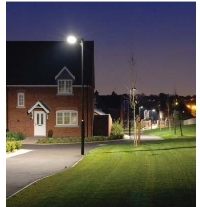
Image showing excessive light spill from a column mounted luminaire – careful luminaire selection and positioning should be used to avoid light trespass such as this.
