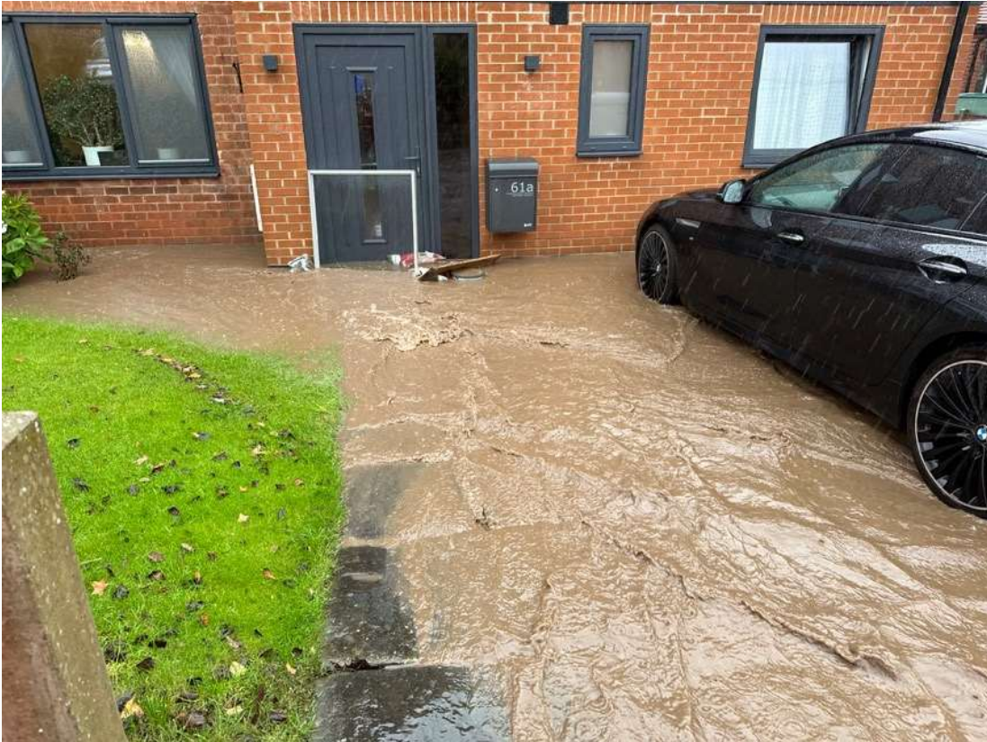
This surface water then further floods properties on Sotheby Avenue and Cardinal Court. Photo from Oct 2023.
