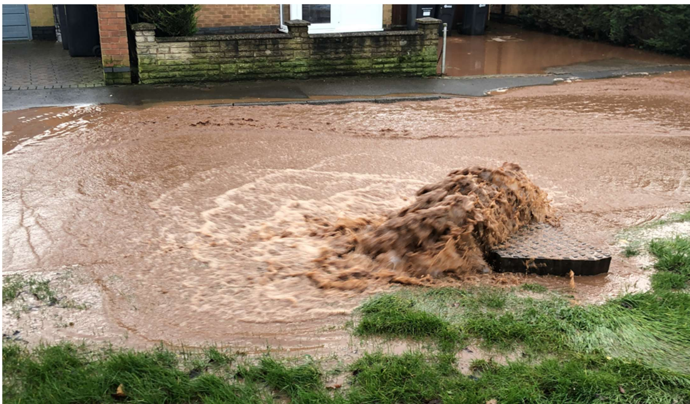
Manhole cover on Newark Road service road lifted off by flood waters. Photo from Feb 2020
