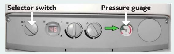
If your boiler has low water pressure, your needle on the right-hand side of the boiler will usually be at 0 or below 1. The display will read **E119**. If this is the case, reinstating the boiler to its correct pressure is simple.
