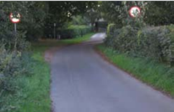
Hedgerows line the roads into Teversal, and help to form a strong, locally distinctive rural character
