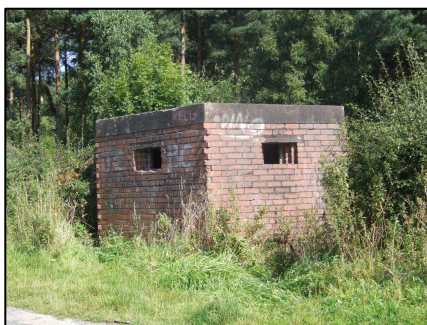
Type 26 WW2 Pill Box , Felley Mill Lane, Underwood; Built as a gun post during WW2 at the junction of Felley Mill Lane North & South.
