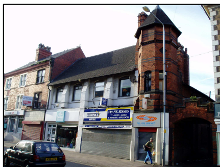
Watson Fothergill Property , High Street, Hucknall; Ornate Victorian property, featuring a tower, designed by the well known Nottinghamshire architect.
