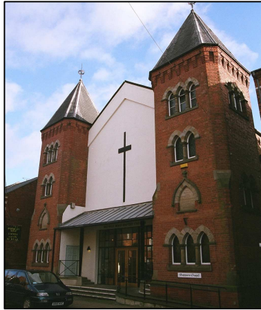
Baptist Church , Watnall Road, Hucknall; Featuring an imposing entrance and twin majestic towers.
