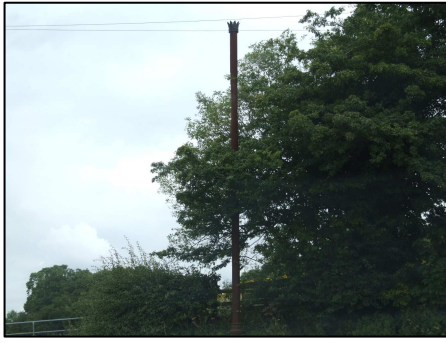
Breather Pole , Dawgates Lane, Skegby (near The Maypole PH): A rare example of the Victorian Sewerage system of Skegby.
