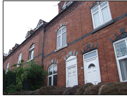
Miners Mid Victorian Terraced Houses , 16-76 Watnall Road: constructed specially for the colliers who worked at the Hucknall collieries and are typically symbolic of the type constructed by mine owners for their employees.
