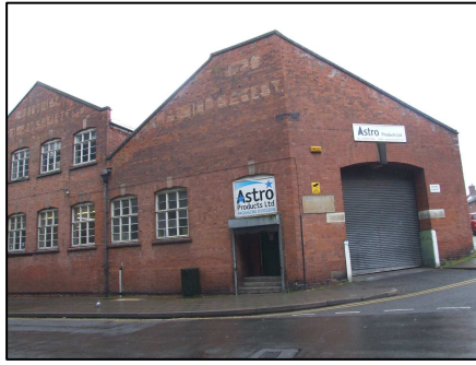
Astro Products , West Street, Hucknall; this was originally constructed as the Co-op Bakery during the mid twentieth century and now used for manufacturing. The original Co-op advertising on the upper walls can still be seen.
