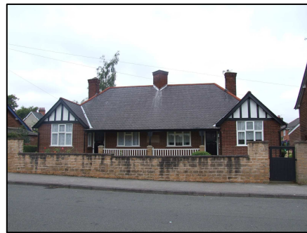
Elizabeth Ann Coupe Alms Houses , 66 & 68 Garden Road, Hucknall; Constructed in 1929 as retirement homes for the poor.
