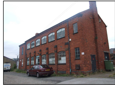
Certa Cito (The Old Forge) , Bolsover Street, Hucknall: Constructed as a hosiery manufacturing building in typical local red brick.
