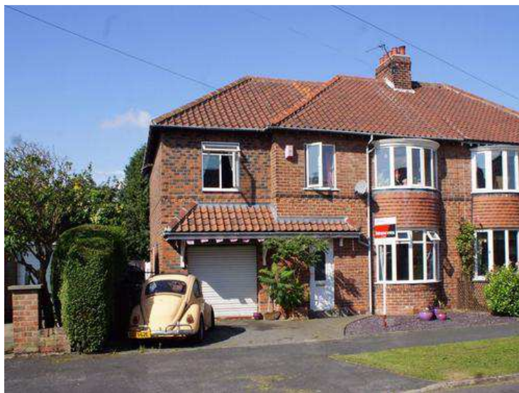
Well designed two storey side extension, with appropriate use of materials
