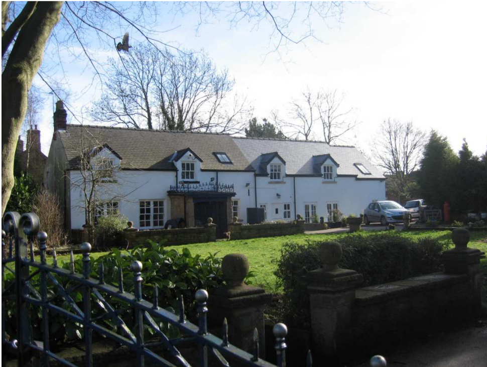
Example of an extension in a Conservation area reflecting the existing dwelling and respecting the character of the area
