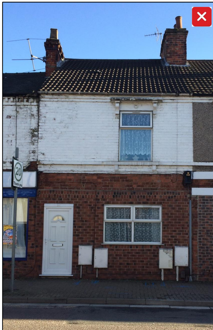
Poorly sited and designed meter boxes can spoil the appearance of the street and the property its self.
