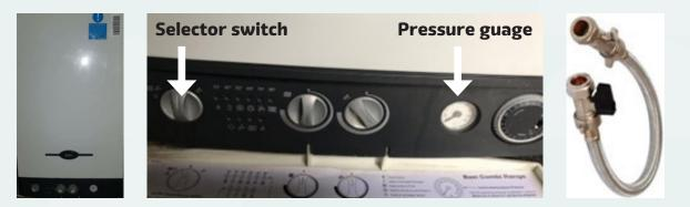
If your boiler has low water pressure, your needle on the right-hand side of the boiler (see picture 2) will usually be at 0 or below 1. The light above number 60 will be flashing, which indicates a pump or low pressure fault. If this is the case, reinstating the boiler to its correct pressure is simple.
