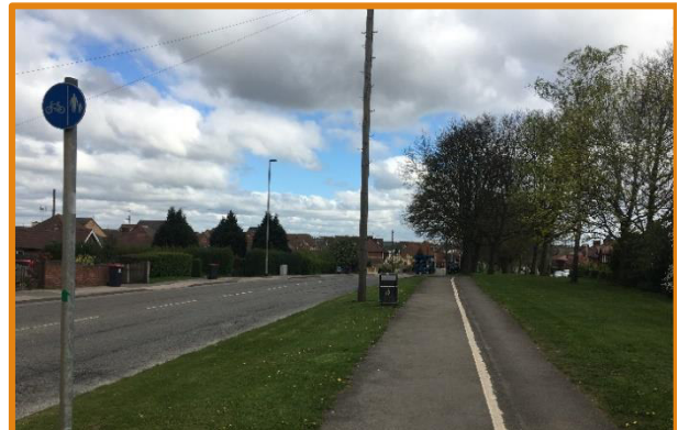
Photograph 7: footways on Kirkby Folly Road/Low Moor Road
